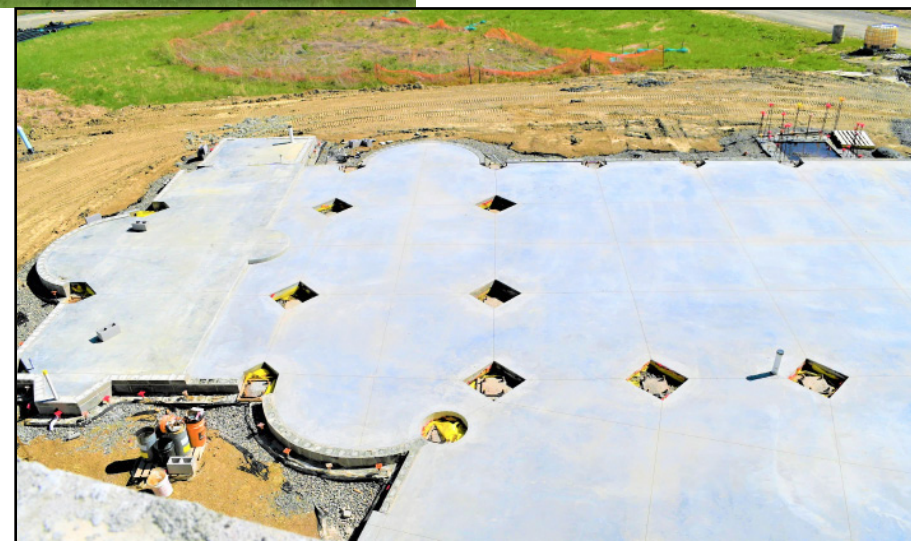
Chapel concrete slab poured
